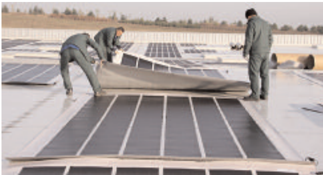
ProLogis Solar Panel installation, Moissey Cramayel, Chanteloup, France
