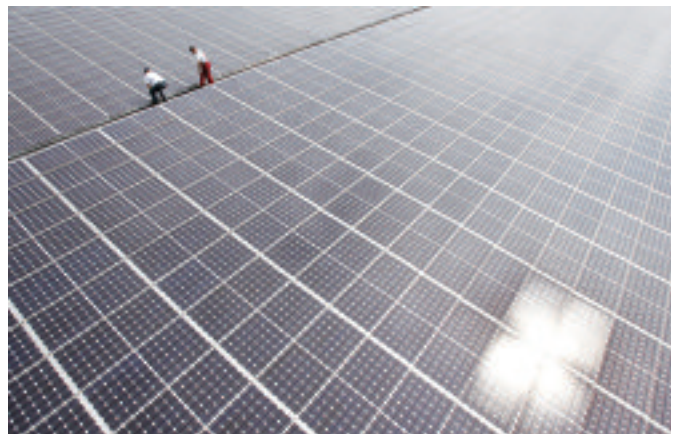
ProLogis-Solar Panels Installed
